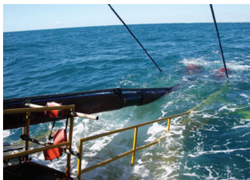
Smart® Band installed on Piggyback Pipelay operation
